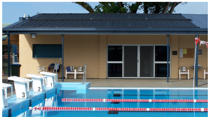
INNISFAIL COUNCIL POOL, QLD
